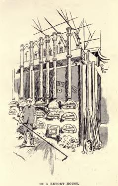
be charged at both ends. They are set side by side, as the illustration shows, and are kept at a red-heat by immense coke furnaces underneath.
