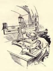
DRILLING HOLES FOR PINS.
